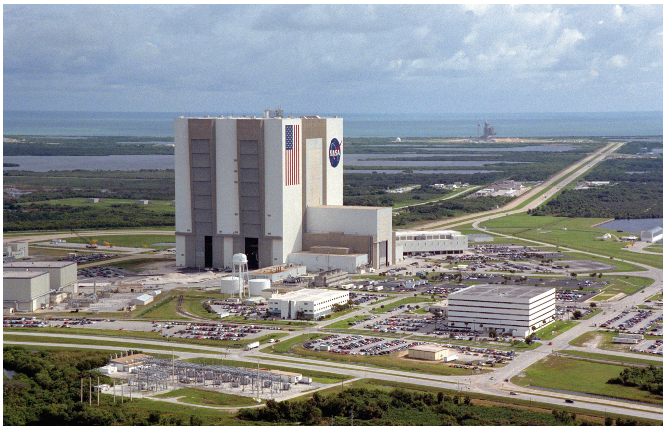
The Vehicle Assembly Building (VAB) at the Kennedy Space Center. One of the largest buildings in the world by volume, the VAB was designed to assemble the Saturn V rocket in its vertical orientation. Photo: NASA
